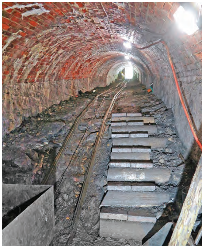
Wallsend Drift: the main haulage adit, looking to surface.
